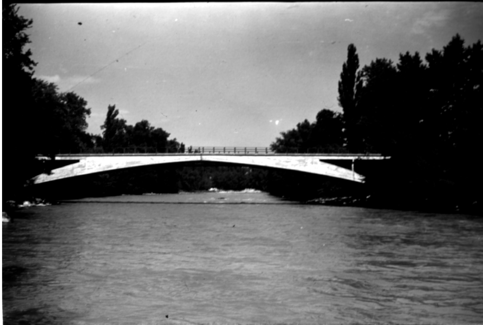
Arve Bridge, 56.0m, 1936
