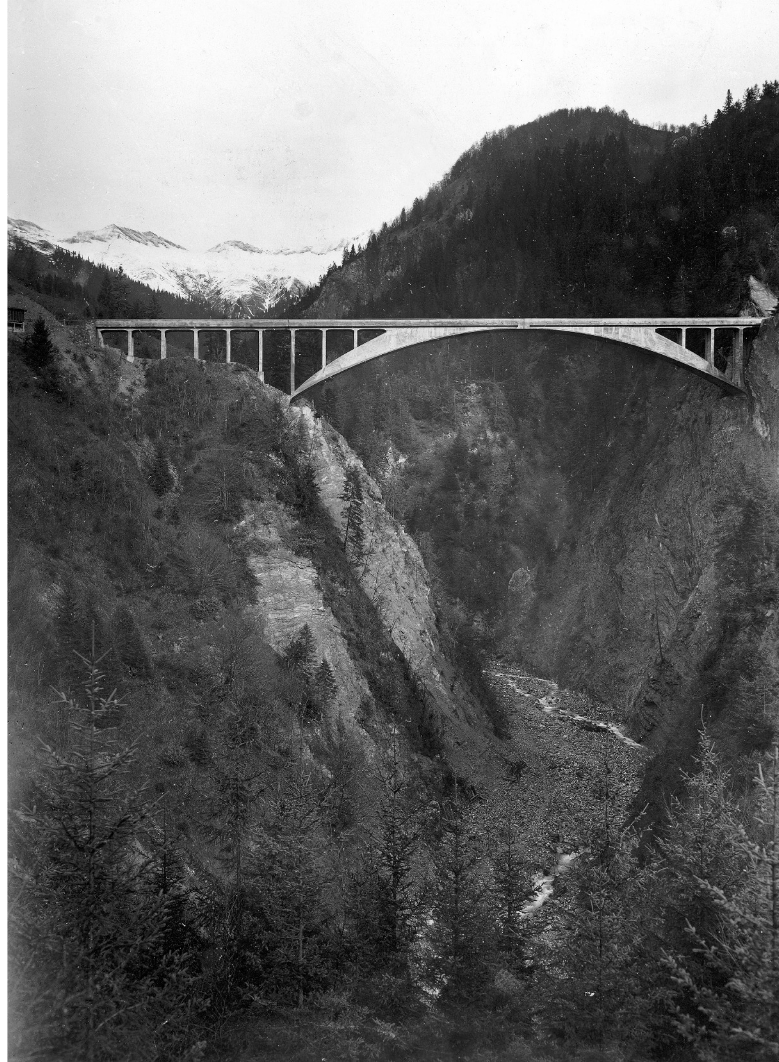
Salginatobel Bridge, 90.0m, 1930
