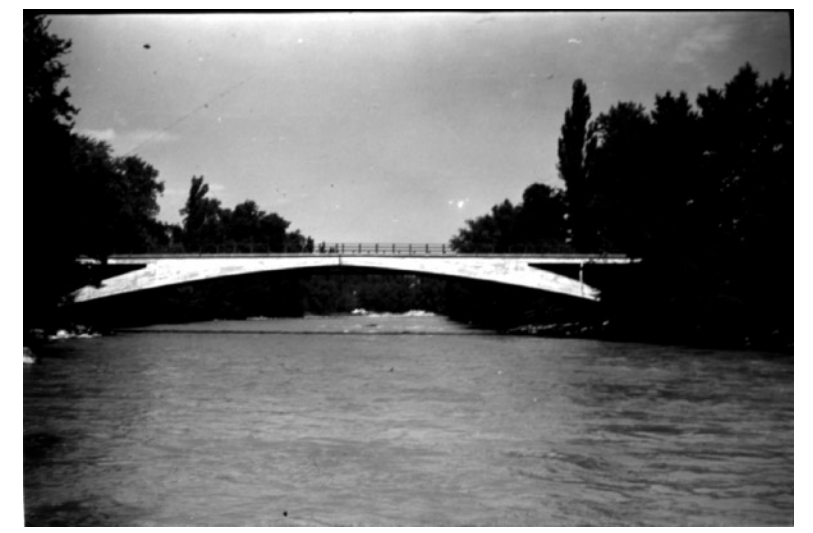
6_Arve-Brücke, Vessy-Genf, 1936, 56.0m
