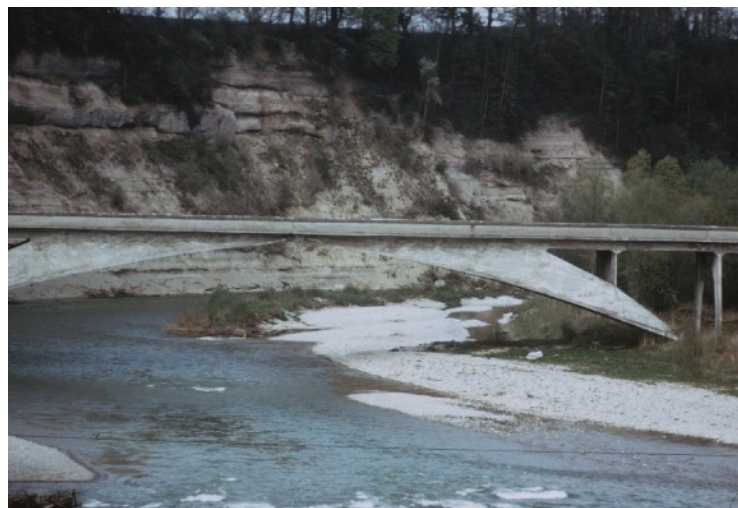
5_Thur-Brücke, Felsegg, 1933, 72.0m
