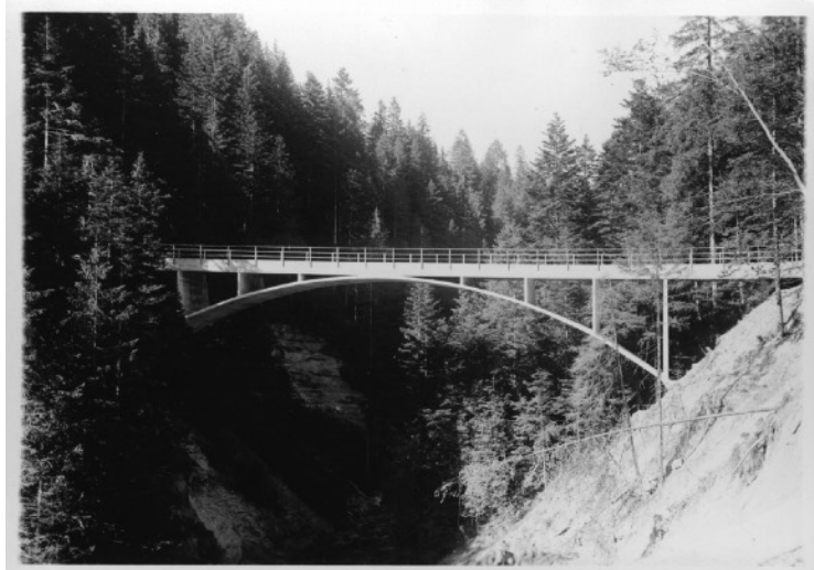
4_Schwandbach Bridge, 1933, 37.4m
